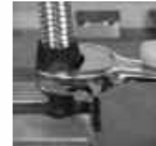
Holding the fitting in the vice jaws, lubricate the nipple and start to thread the socket onto the fitting taking care not to cross thread.
